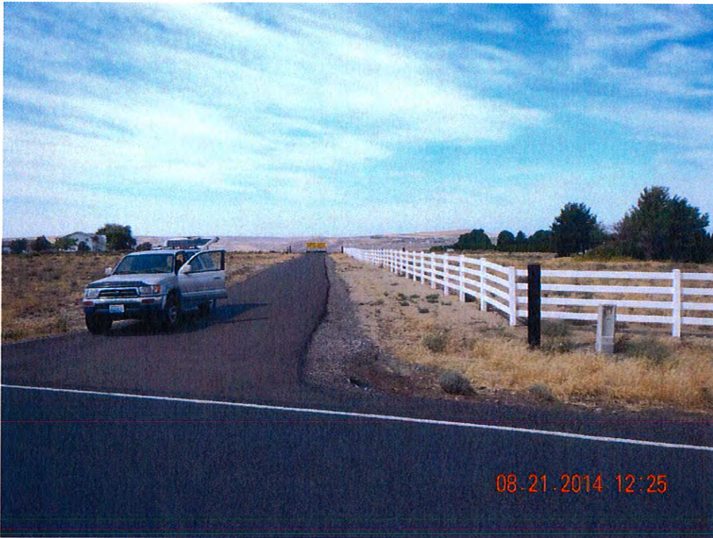
7. Looking west from the proposed new power pole location and proposed underground utility route.
