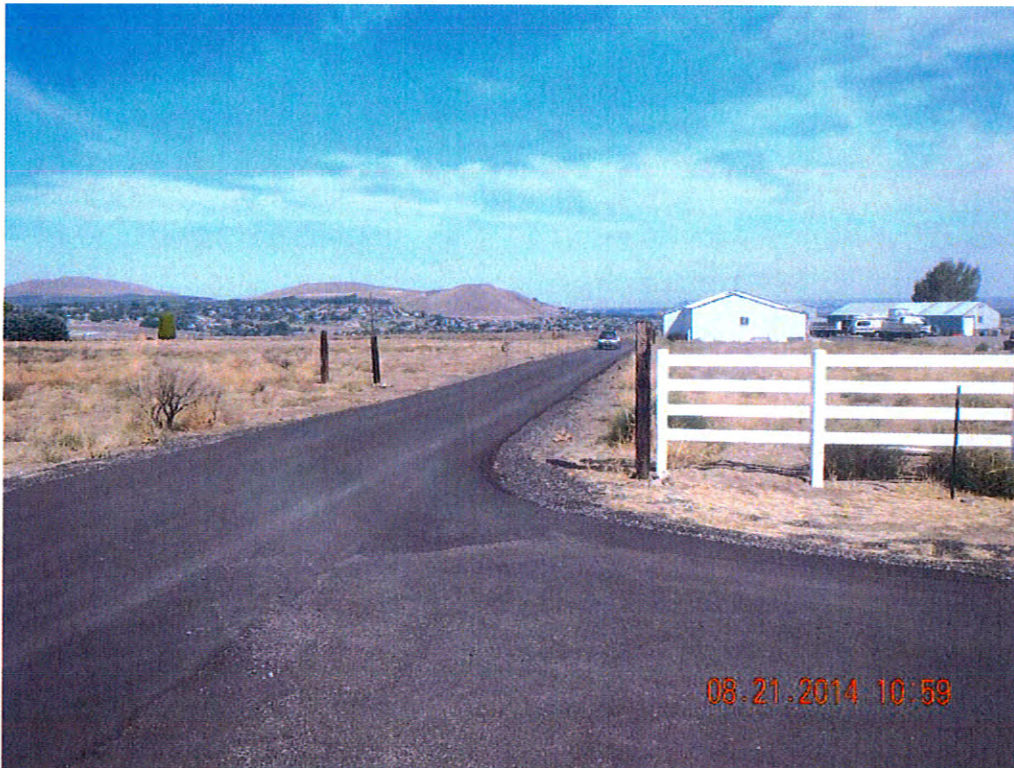
8. Telecommunications and power is proposed to be routed underground to the proposed lease area.
